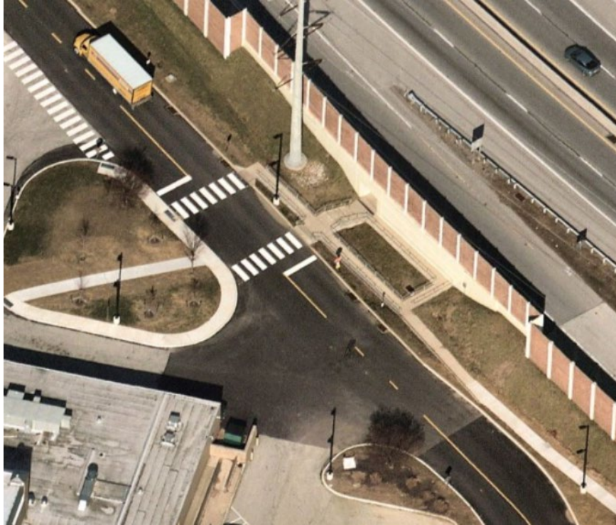
Crosswalks improved at pedestrian path connecting to middle school
