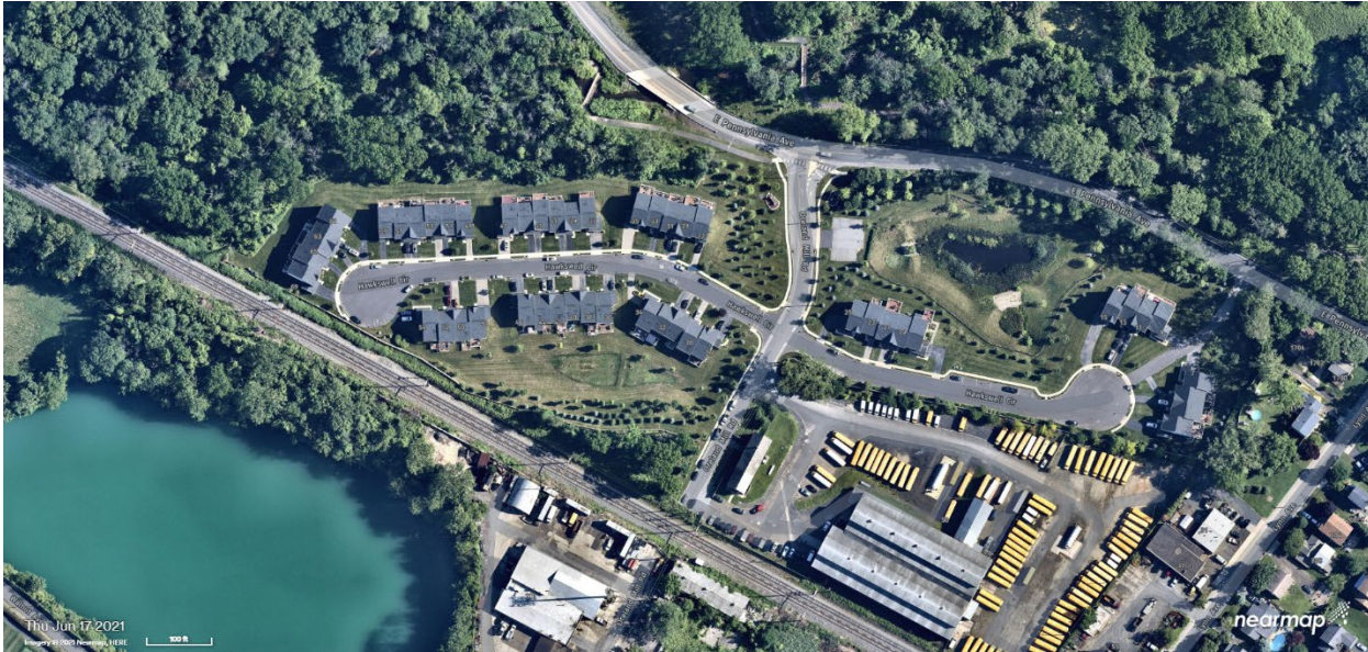
Aerial View of Site
