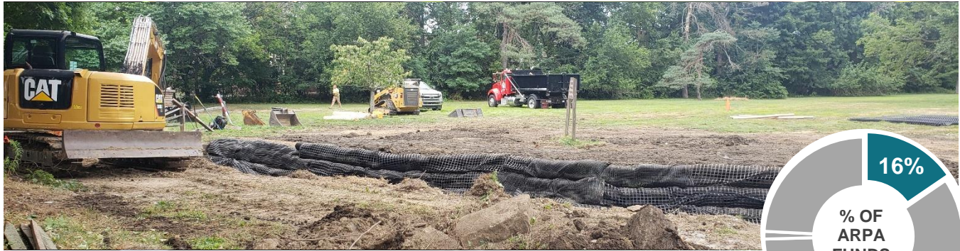
STREAMBANK STABLIZATION AT MERMAID PARK
