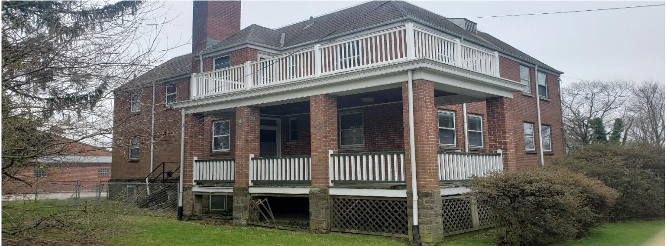
FORMER RECTORY AT 1200 WILLOW GROVE AVENUE
