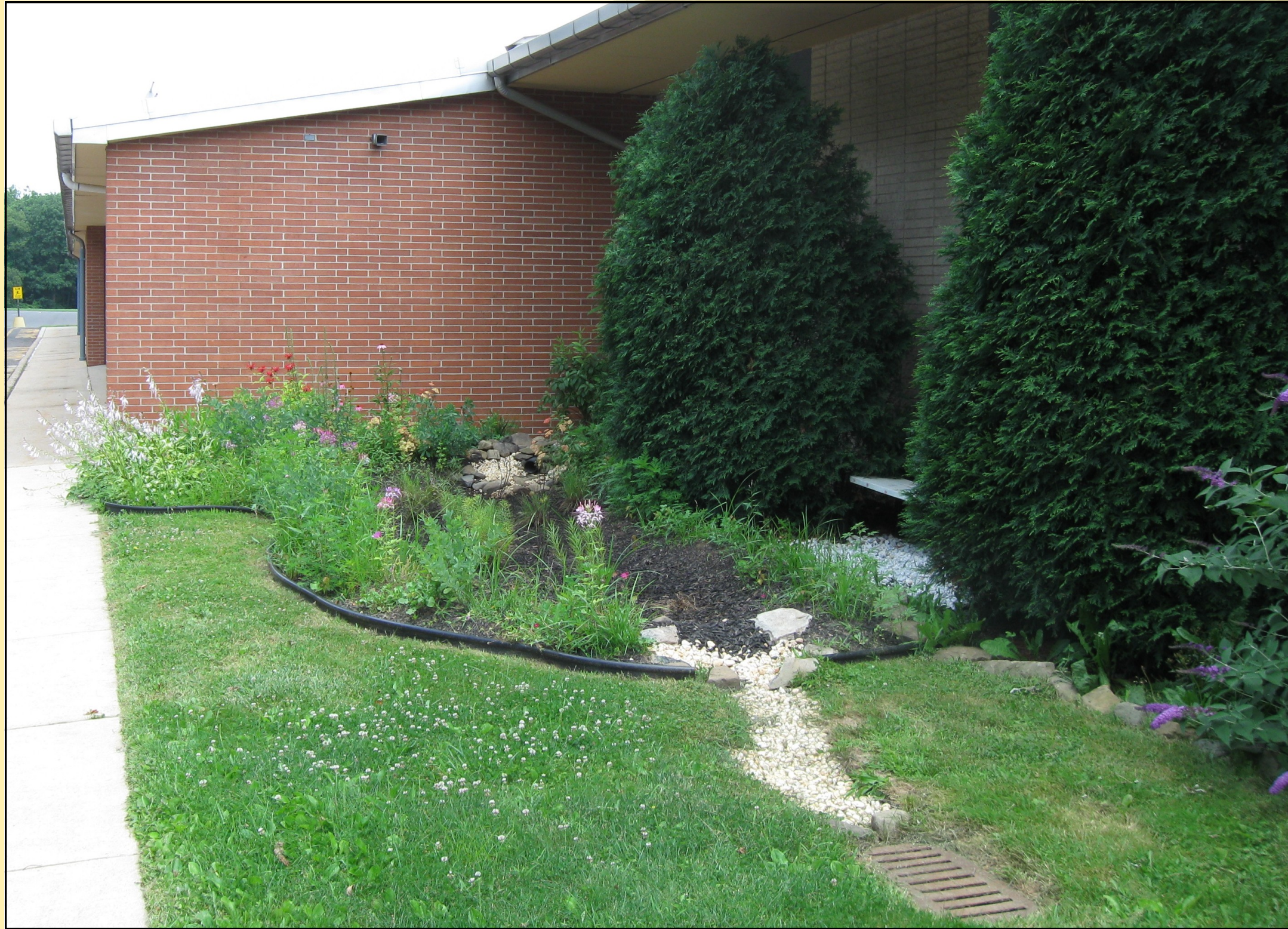
Rain gardens can be used to collect water from rooftops as shown above at Blair Mill Elementary School in Horsham Township, Montgomery County.
