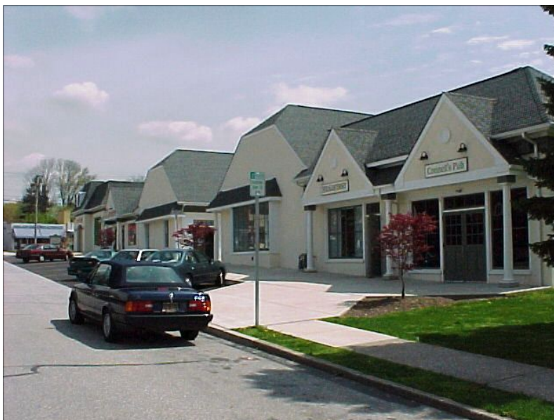
The Oreland Shopping Center would benefit from adequate tree cover.
