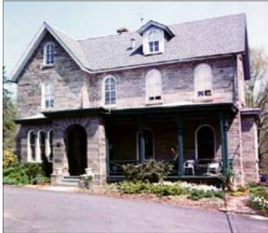
Keystone House, Built 1867
