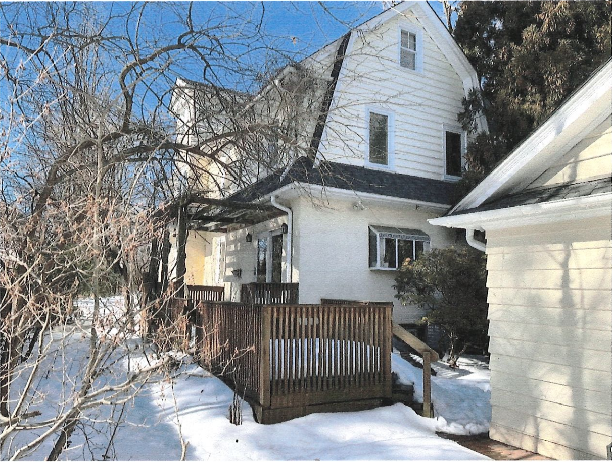
2) Side yard view looking toward house and existing rear deck.
