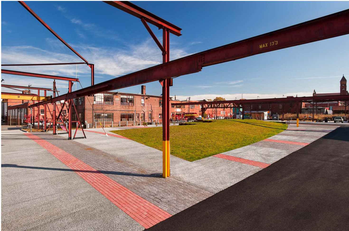
The Steel Yard, RI (KMDG)
