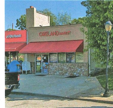
FRONT VIEW OF BUILDING
