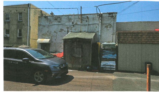
REAR YARD LOOKING AT BUILDING
